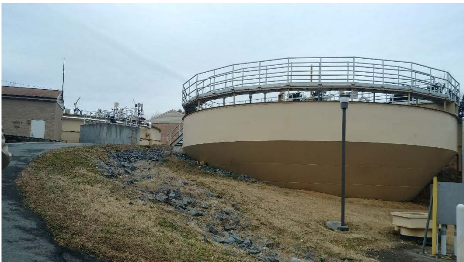
La Plata WWTP, Charles County, MD
