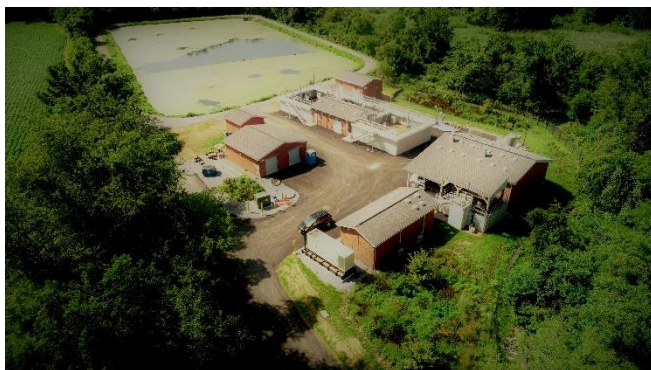
Galena WWTP, Town of Galena, Kent County, MD.
