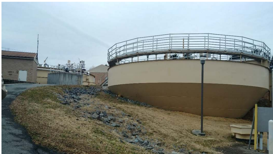
La Plata WWTP, Charles County, MD
