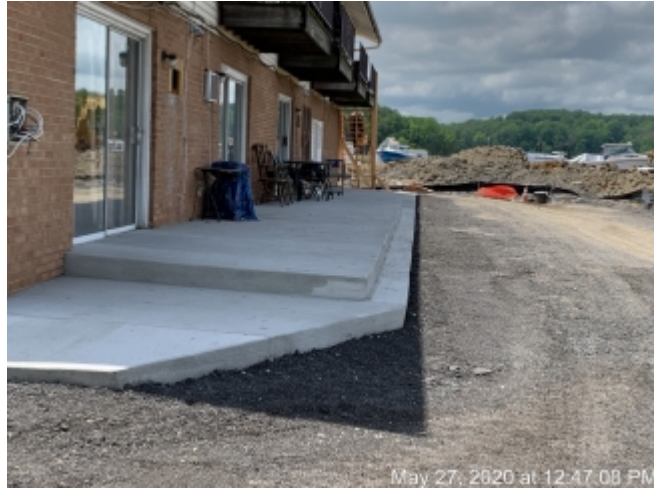
Uploaded on: 05/28/2020 - May 27, 2020 New sidewalk - North Side
