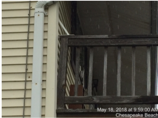
Uploaded on: 06/13/2018 - May 18, 2018 Railing Pulling Away
