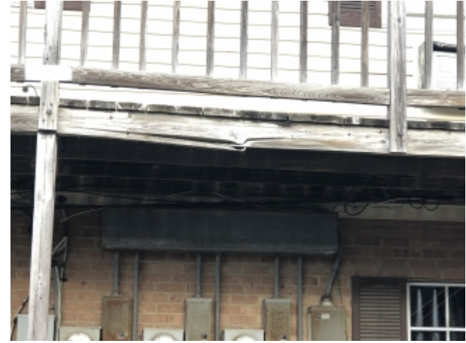
Uploaded on: 01/06/2020 - Decking 4 1.3.2020
