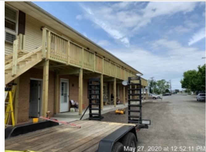
Uploaded on: 05/28/2020 - May 27, 2020 New Decking South Side
