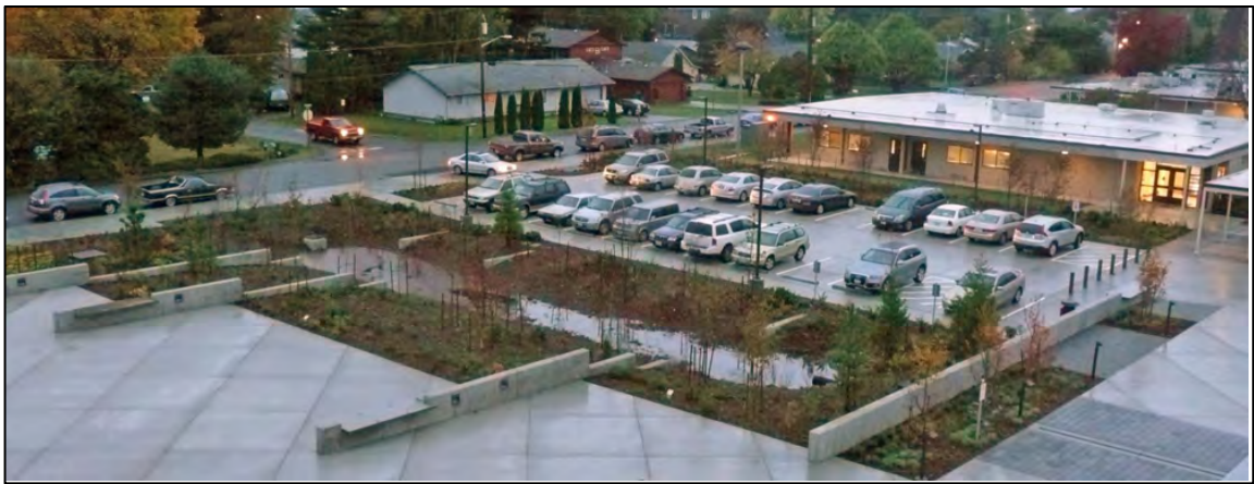
Figure 28: Image of parking lot providing stormwater management.
