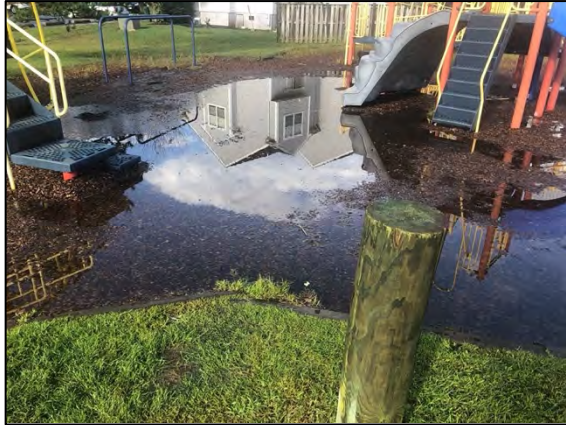
Figure 12: Standing Water at the Tot Lot at Kellam's.
