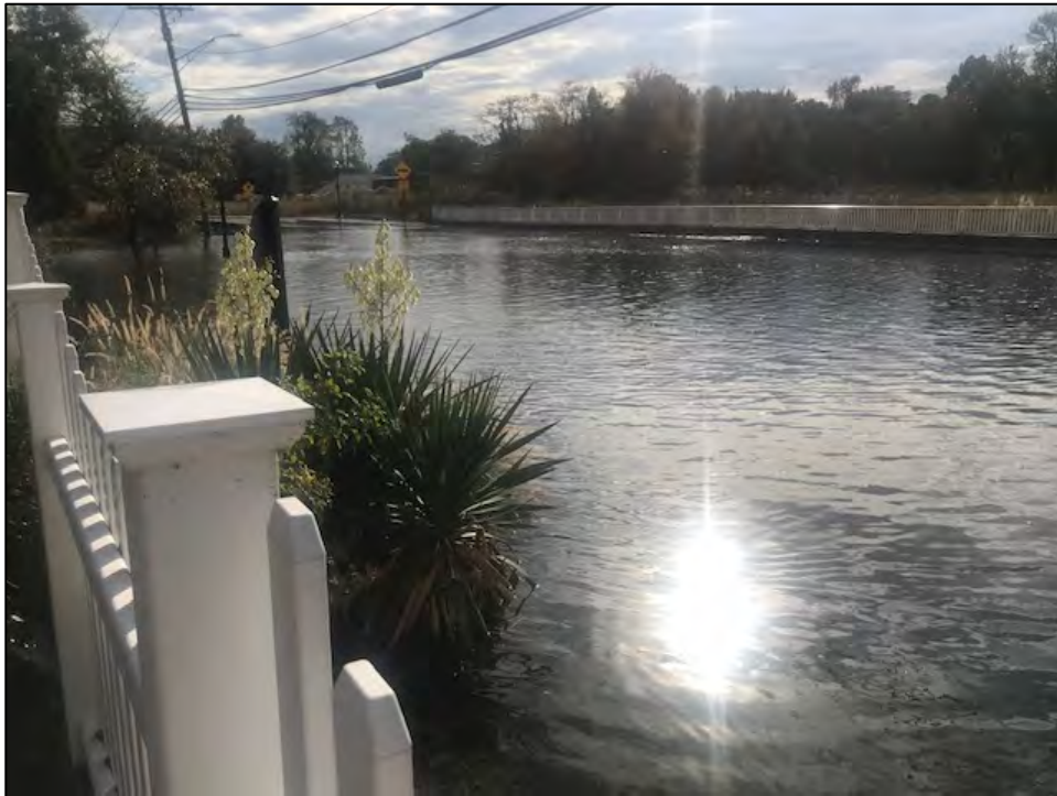
Figure 15: View from Sea Gate community along MD 261 frontage looking west toward the sidewalk railing on MD Route 261 which is underwater following the un-named high tide event on October 12, 2022.
