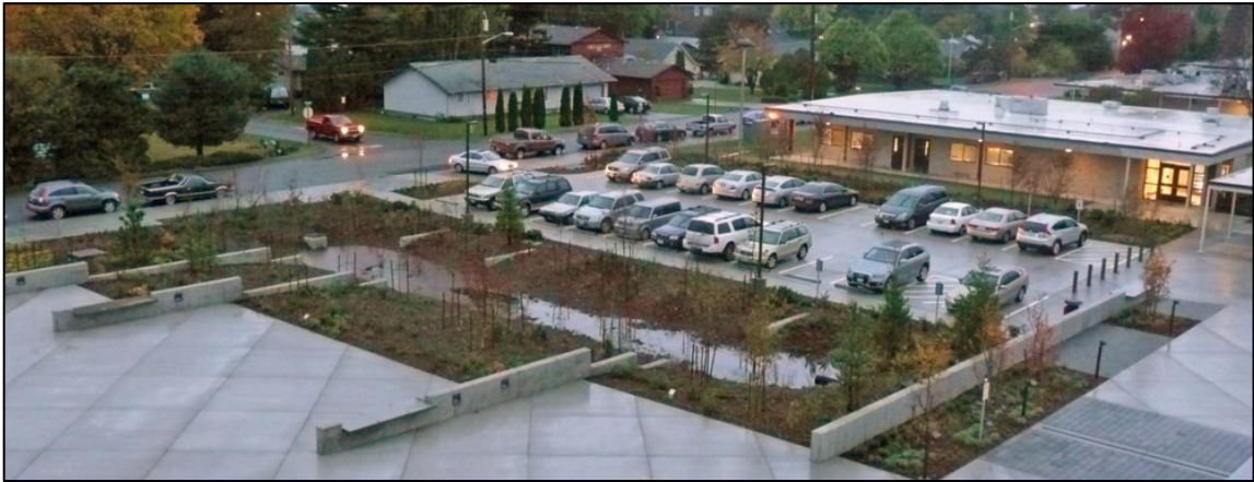
Figure 27: Image of parking lot providing stormwater management.
