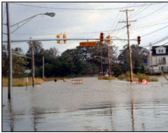
Figure 1: 2003 Photo Following Hurricane Isabel. MD Route 261 (Bayside Road) at the entrance to the Volunteer Fire Company, looking north.
