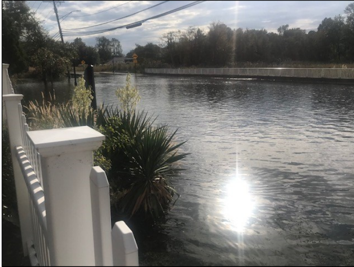
Figure 1445: View from Sea Gate community along MD 261 frontage looking west toward the sidewalk railing on MD Route 261 which is underwater following the un-named high tide event on October 12, 2022.
