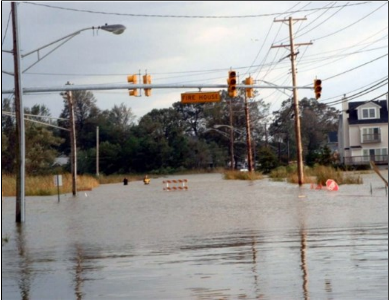
Figure 1: 2003 Photo Following Hurricane Isabel. MD Route 261 (Bayside Road) at the entrance to the Volunteer Fire Company, looking north).
