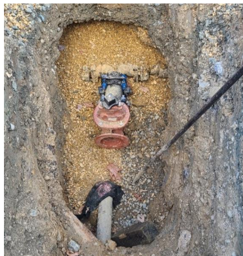
Picture 6 Administration Building Tie-In
