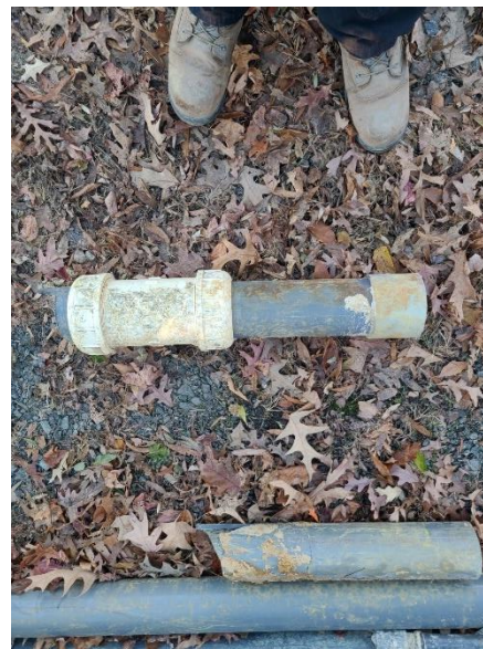
Picture 3 Compression Coupling Removed
