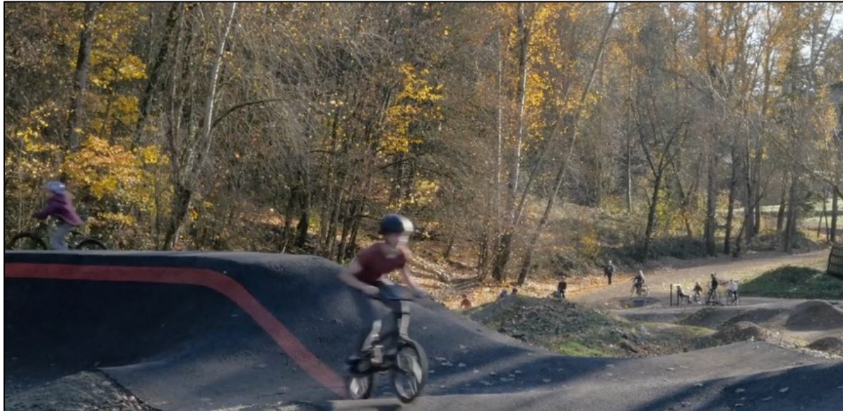
Figure 35: Source, American Ramp Company. A potential recreational use for the landforms that would be established to help protect Kellam's Recreational Complex.
