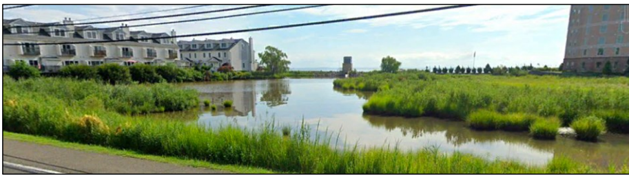
The floodgate, with its revetment and causeway, were intended to prevent storm surge from entering the wetland and flooding the northern part of Town, including Seagate and MD Route 261 9 . However, the floodgate is in a permanently open position, so it does not operate to prevent tidal flooding. Figure 15 shows that MD Route 261 was inundated by the October 2022 unnamed tidal event that occurred without precipitation.
