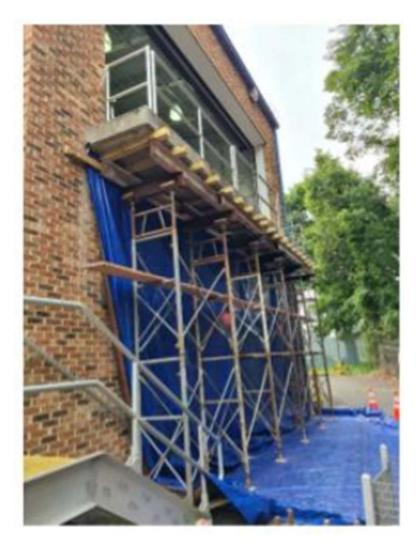
The overhang was cut flush to the wall, and the removed concrete was lifted from the scaffold using a forklift. Exposed reinforcing bars were ground back to the concrete and corrosion inhibiting spray was applied to the exposed metal. A skim coat of cement was applied to the face of the concrete and the existing handrails were reinstalled.
