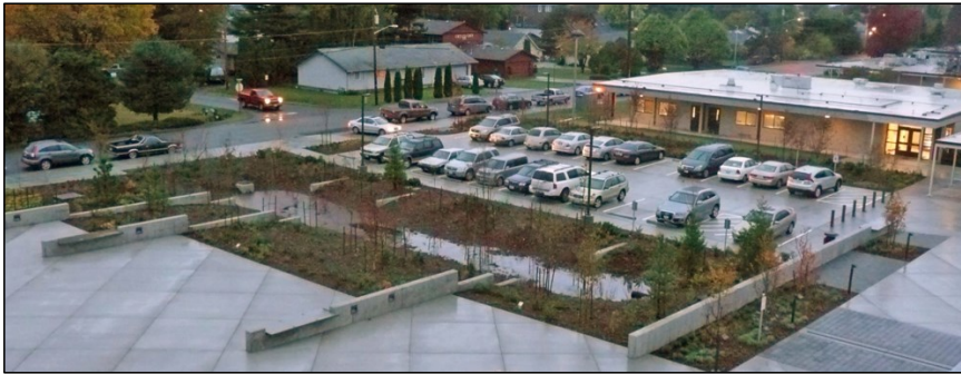
Figure 28: Image of parking lot providing stormwater management.
