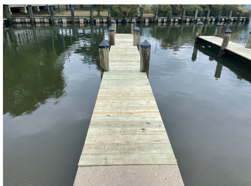
New ramp decking at the Town boat ramps
