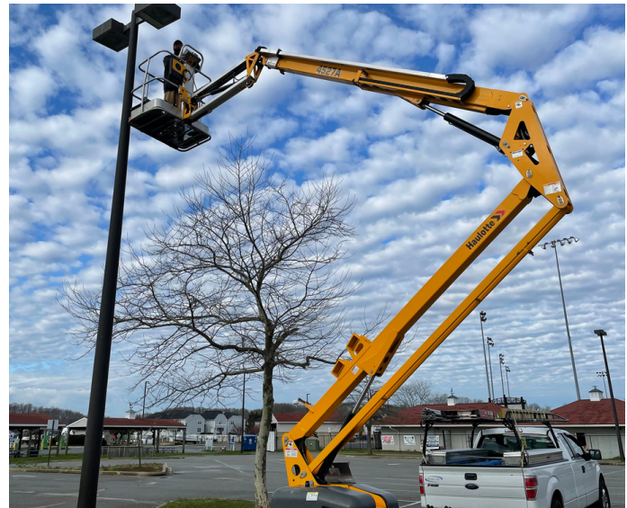
Upgraded Lighting at Kellam's
