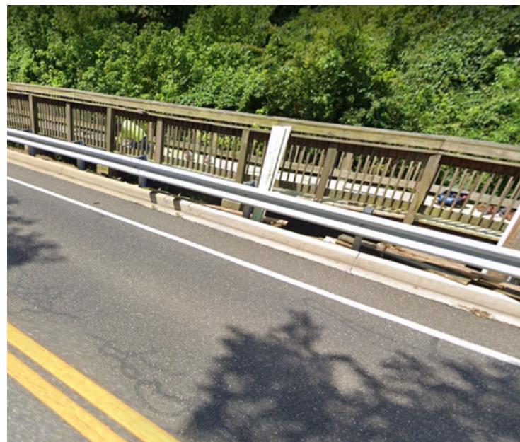
New decking on RT 261 boardwalk
