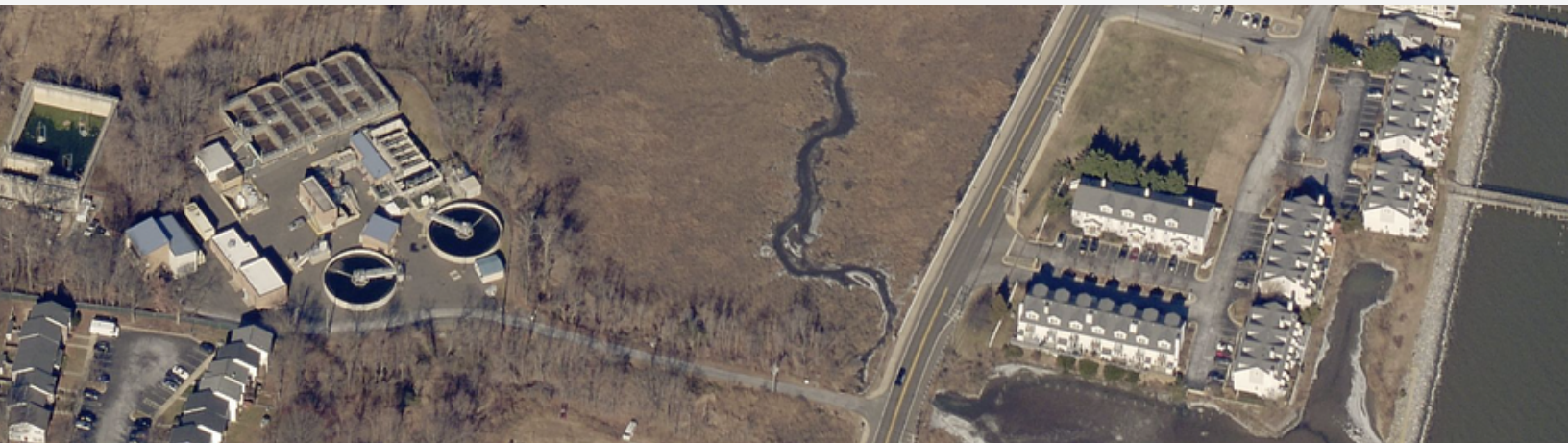
2022 Aerial imagery of the CBWRTP Treatment Plant
