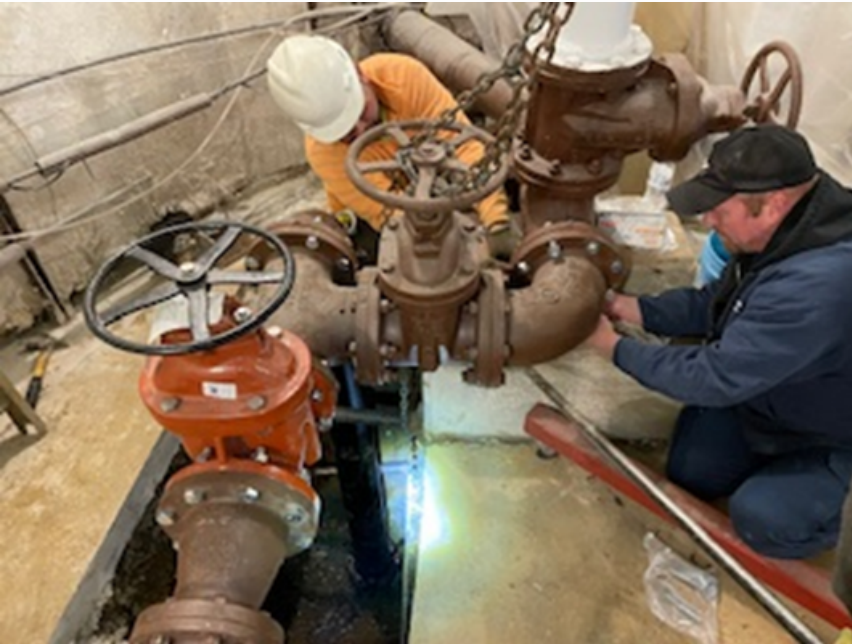
William Varner, Town of Chesapeake Beach Public Works staff working on the replacement of the well pump and valves at Richfield Station Water Tower
