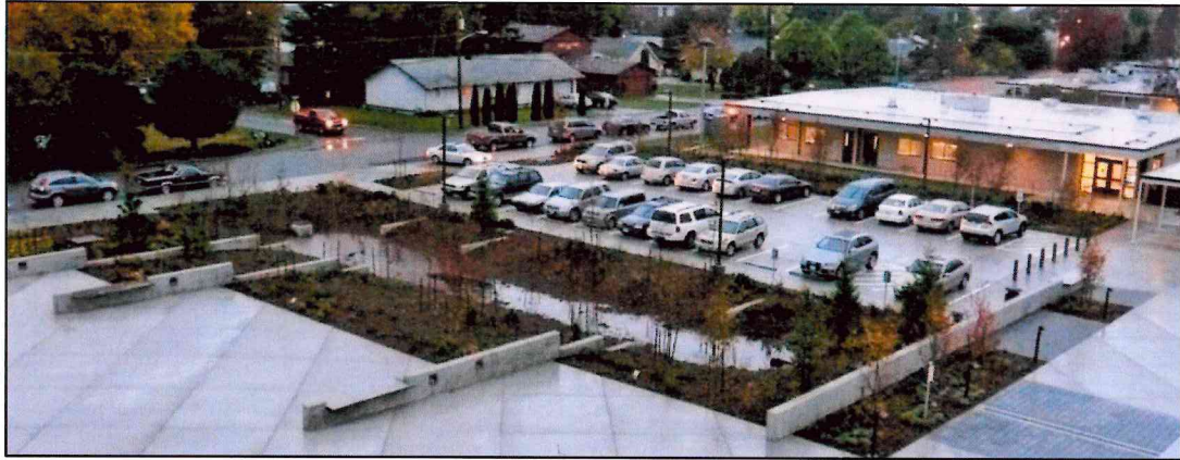
Figure 19: Image of parking lot providing stormwater management.
