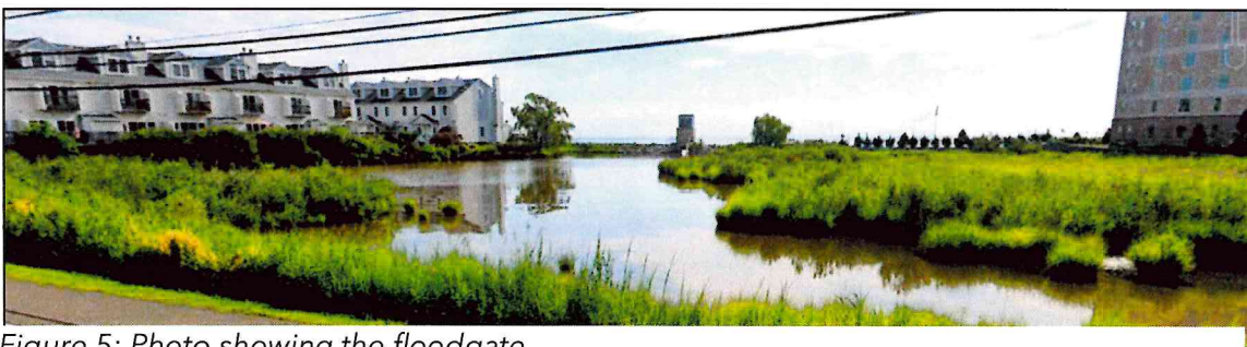
Figure 5: Photo showing the floodgate.
