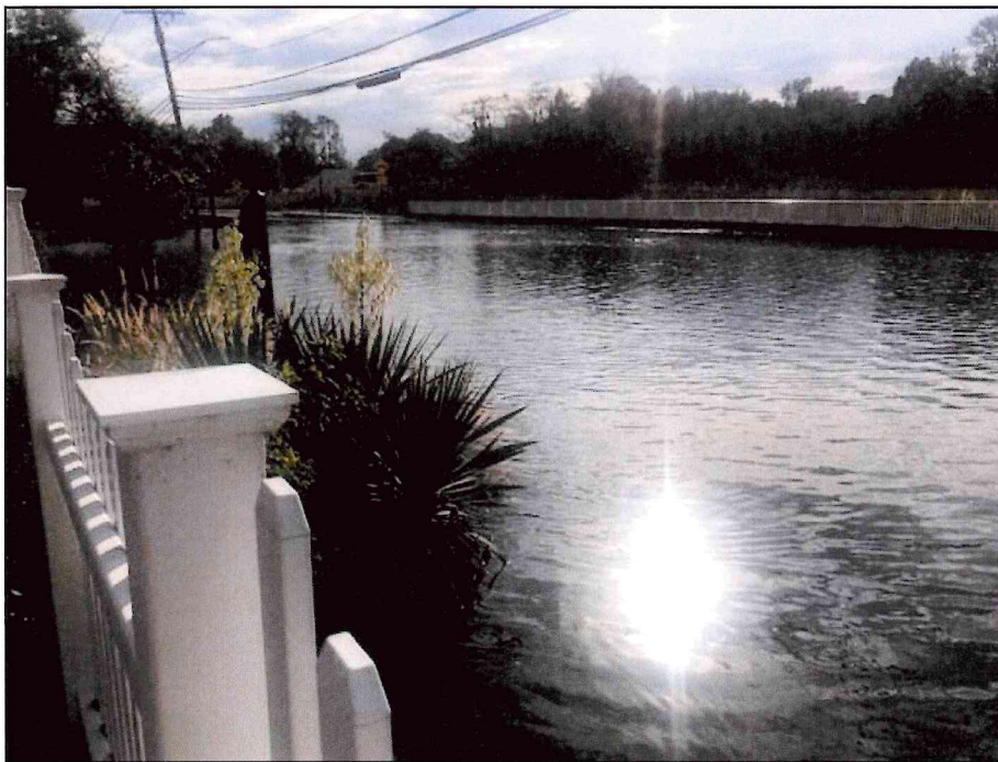
Figure 6: View from Sea Gate community along MD 261 frontage looking west toward the sidewalk railing on MD Route 261 which is underwater following the un-named high tide event on October 12, 2022.
